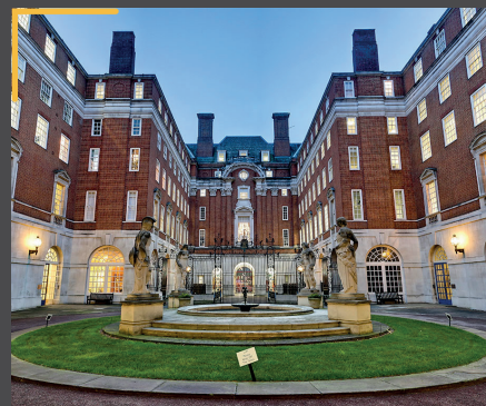
Installed in: British Medical Association House, UK
