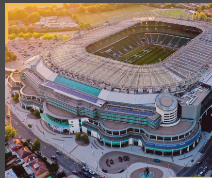
Installed in: Twickenham Stadium, UK
